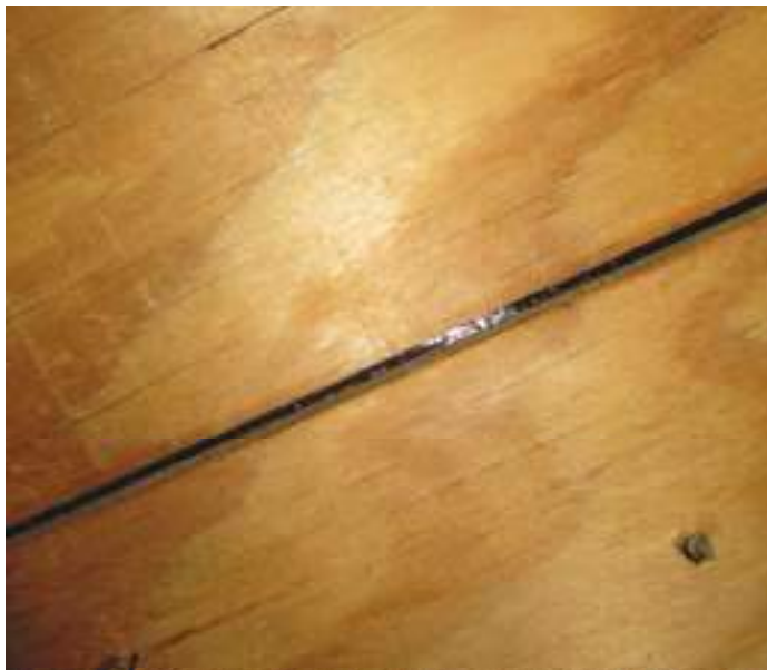
SWR installed under the metal panels
